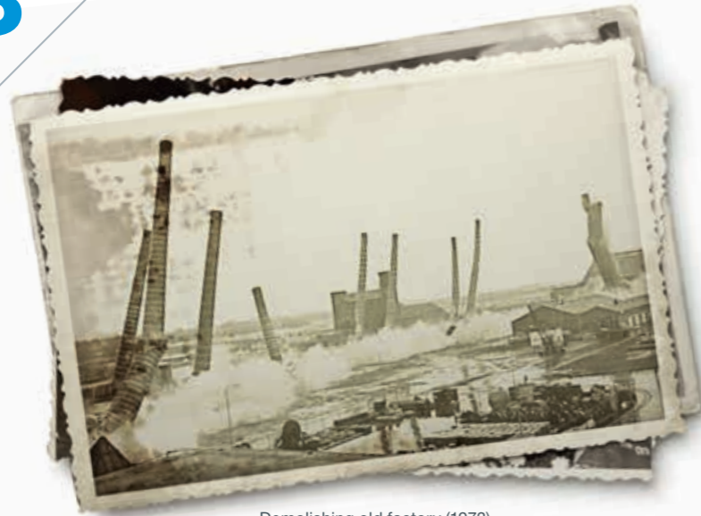
Demolishing old factory (1973)
